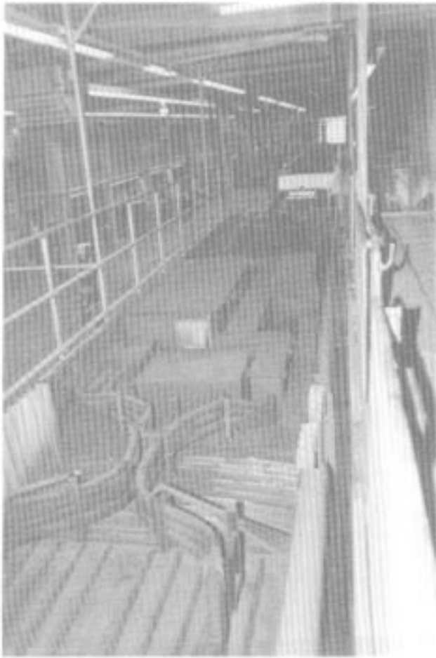
Figure 70. Kassel maintenance shop (photo—showing access to roof equipment).
