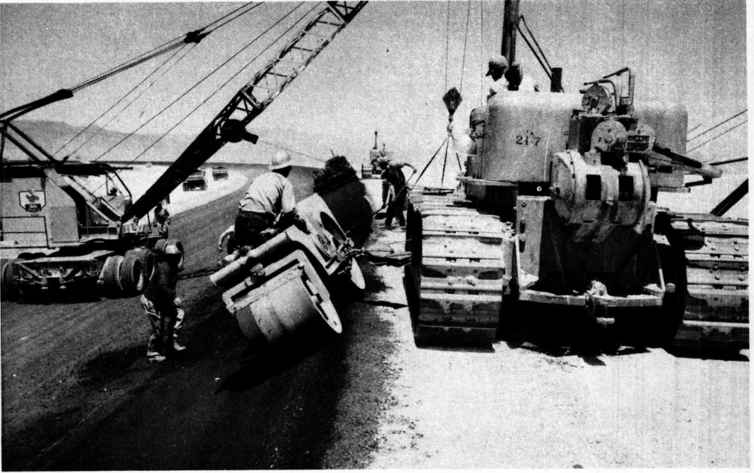
Figure D-3. Paving superelevation - Ford Arizona track.
