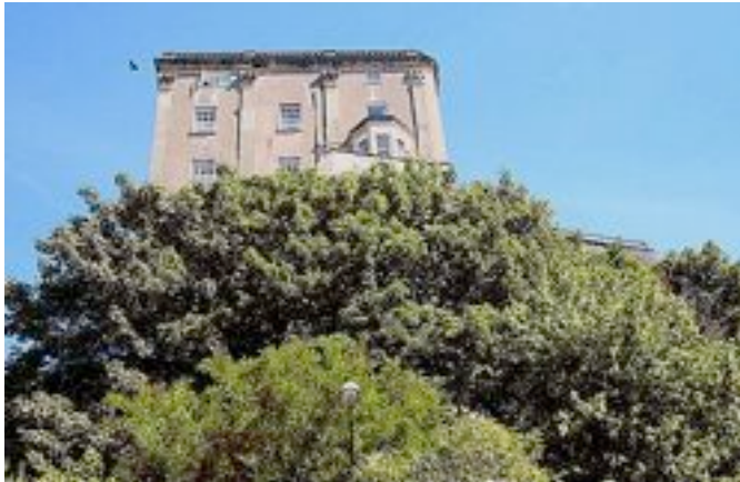
Ap. 1. "Watts' Folly", Clifton, Bristol. William Watts lost his fortune in the construction of this high retaining wall.
