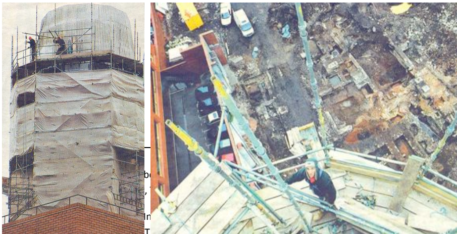
Figures 5, 6. Restoration works in the shot tower.©Evening Post. 26 January 2002.
