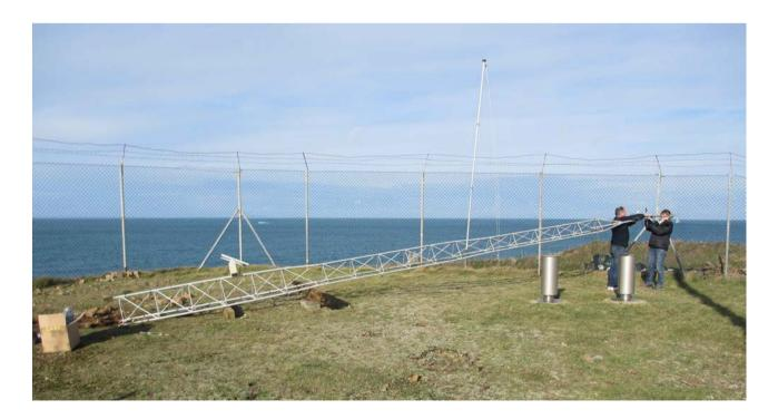
Guernsey Met Office staff lower a 10 metre wind mast at Chouet in order to service and maintain the instrumentation. The wind data from this installation is used for research into the island's potential for generating electricity from wind power and is passed on to the Department of Commerce and Employment. Photo credit: Martin Crozier
