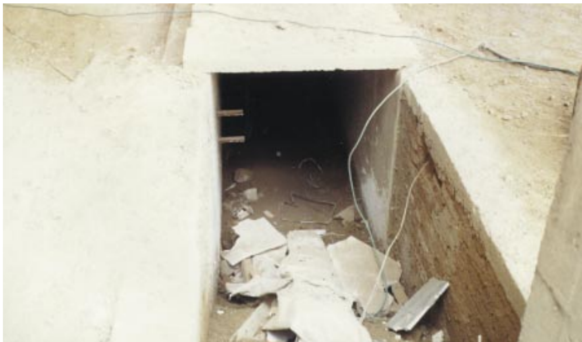
At the Taiyuan space launch center, underground steam and electrical access tunnels measuring three feet by five feet snake beneath and through buildings where U.S. satellites are prepared for launch.
