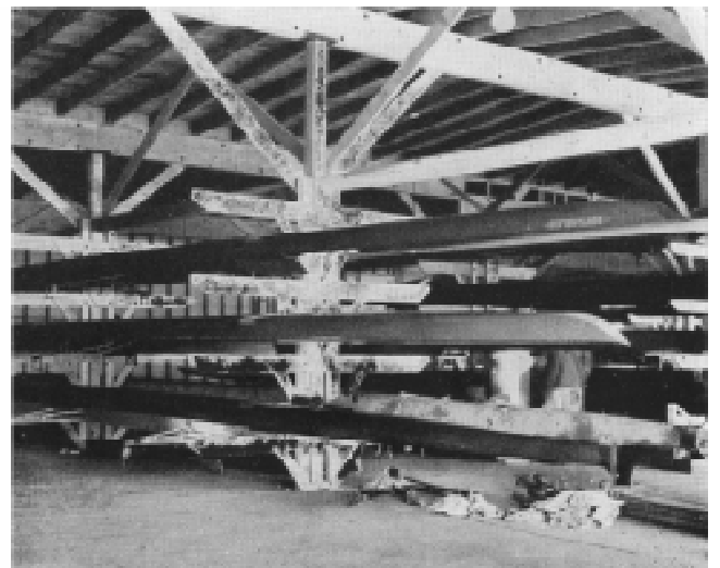
VIEW INSIDE BOATHOUSE
