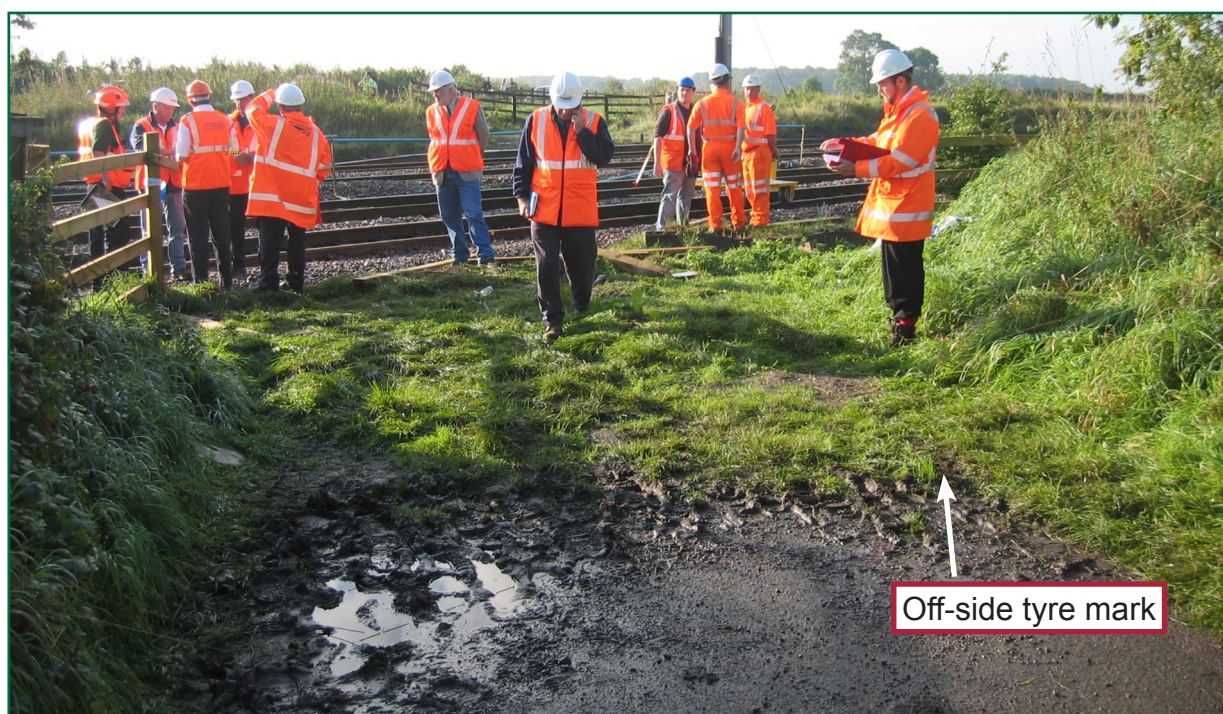
Figure 2: The site of the damaged fence
