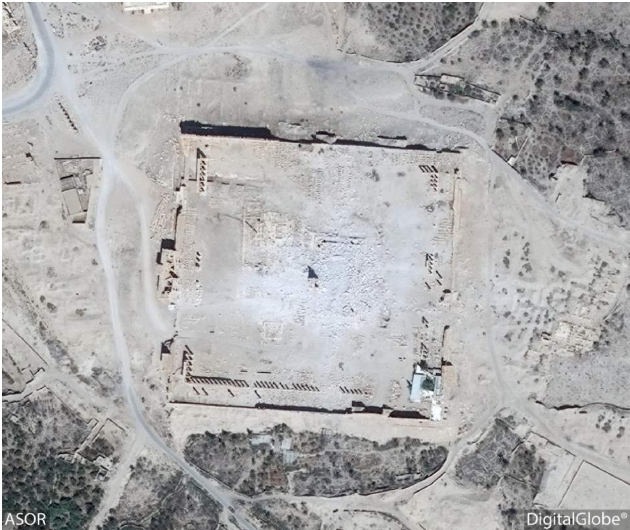
Temple of Bel with visible damage (Digital Globe; September 2, 2015)
