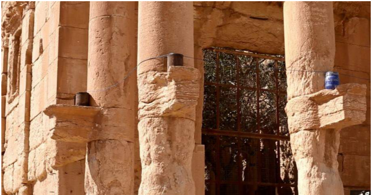
Baalshamin Temple, placement of explosives (ASPA; August 23, 2015)
