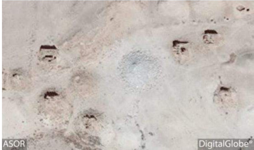
The Tower Tomb of Kithoth with visible damage (Digital Globe; September 2, 2015)
