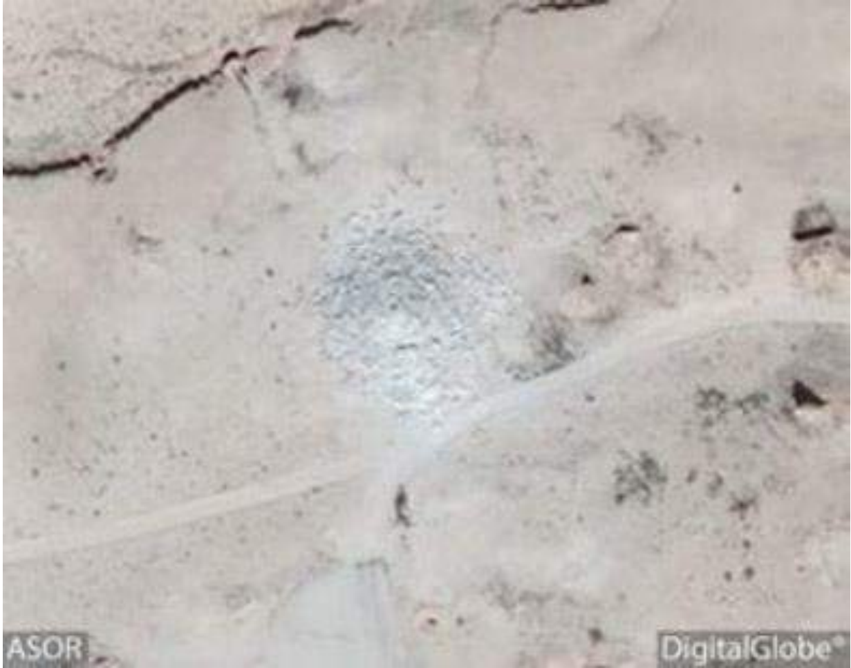
The Tower Tomb of Elahbel with visible damage (Digital Globe; September 2, 2015)
