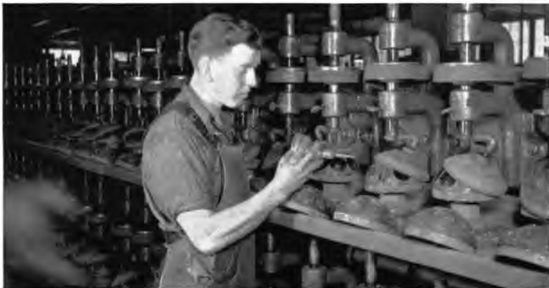
The lenses are ground by means of corundum and water, and the polishing is done with felt-covered tools, using rouge and water.
