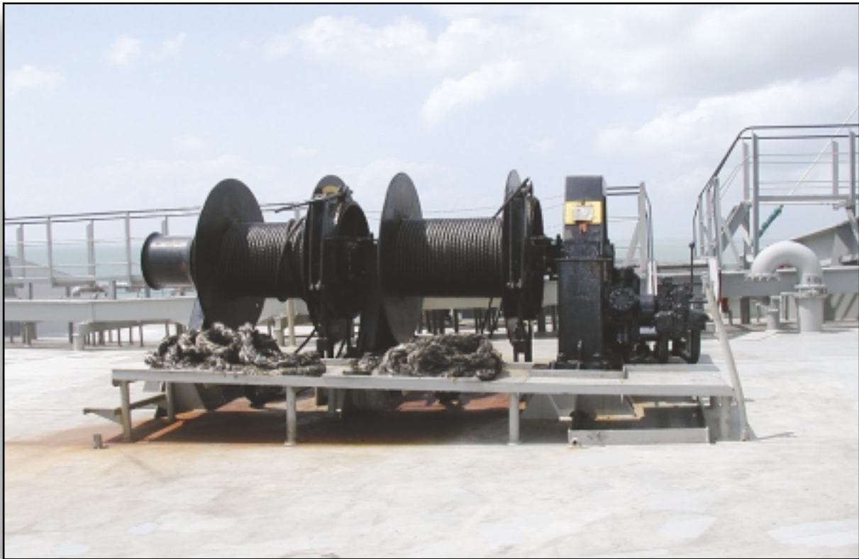
Figure 3.13 – Deck Mounted Reeled-Stowage Mooring Winches
