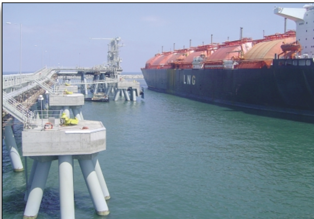
Figure 3.1 – LNG Carrier Approaching the Berth at Cove Point
