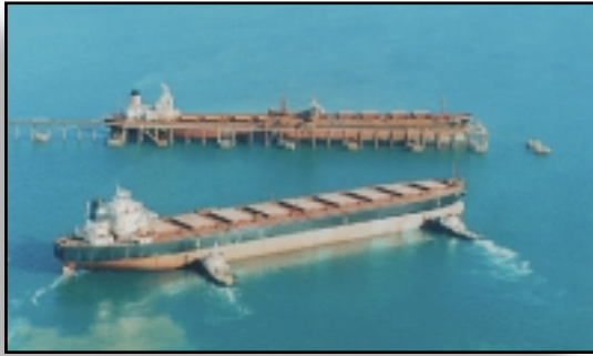
Figure 3.34 – Bulk Carrier Docking Using Laser Docking System
