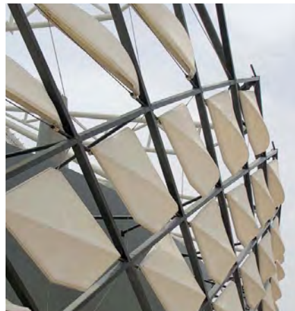
Above left: The angle of Hazza Bin Zayed Stadium's façade panels adjust to meet requirements for shading, airflow and aesthetics (see p. 32).
