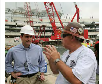
Mark Tamaro of Thornton Tomasetti (left) and Mike Davis of Bosworth Steel Erectors, Inc. on the site of Nationals Park in 2007 (see p. 40).
