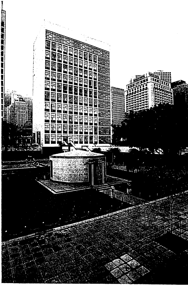
The High Block Building and the shrine in the Memorial Garden
