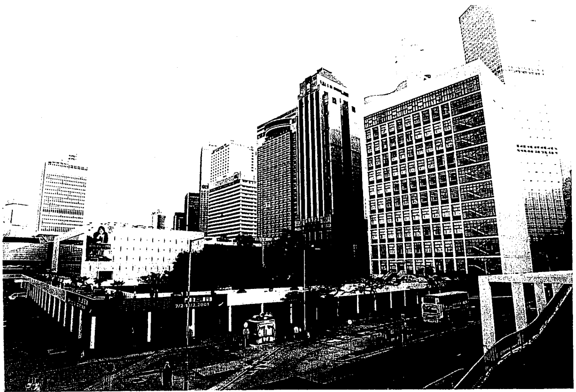
The High Block and the western wall planned to be demolished
