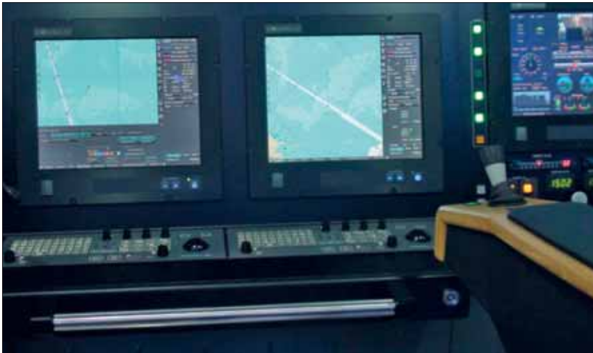
Fig. 5. Control station of a ship
