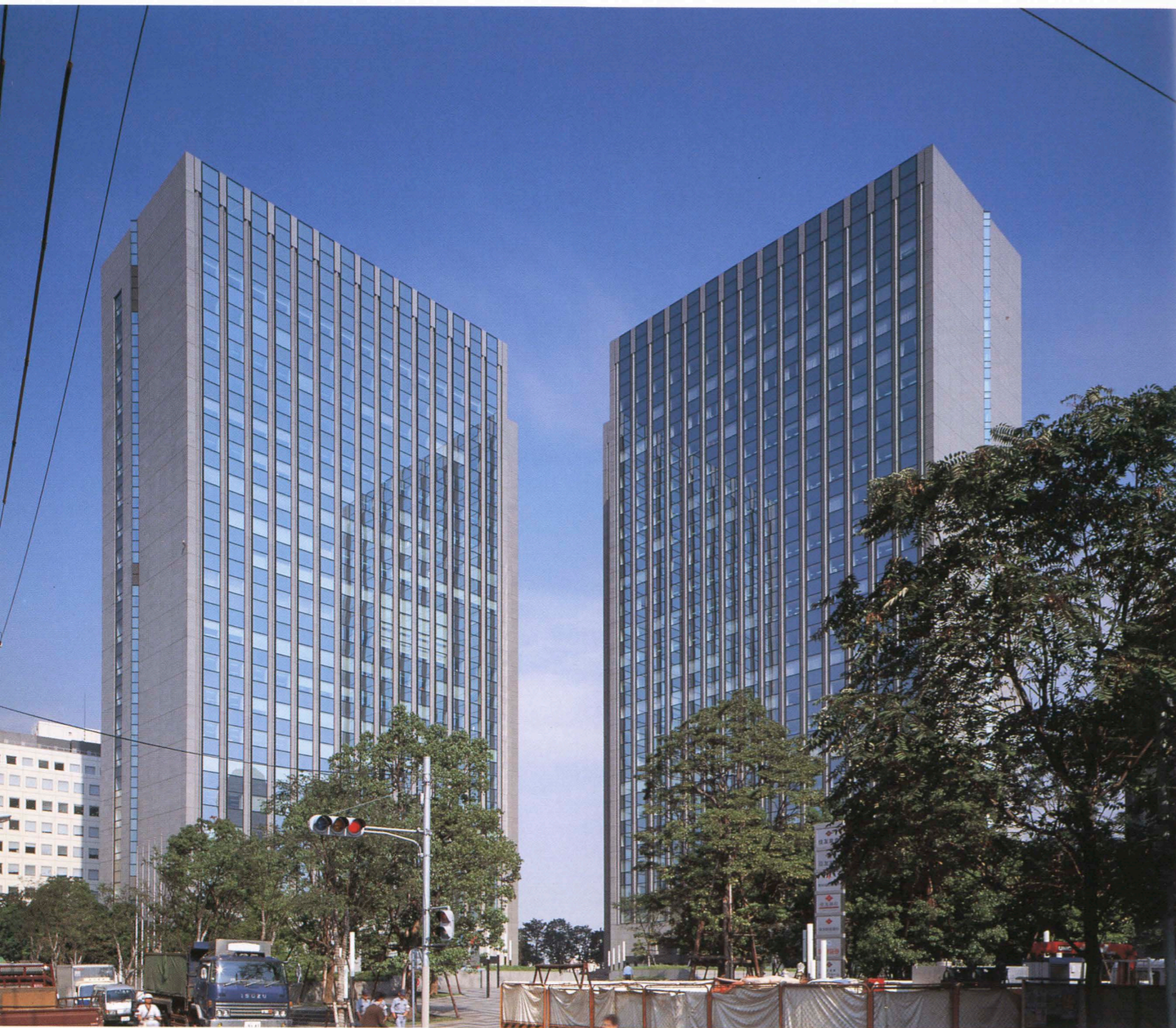
▲面側外観 West side.
