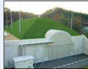
Securing ammunition storage facilities
