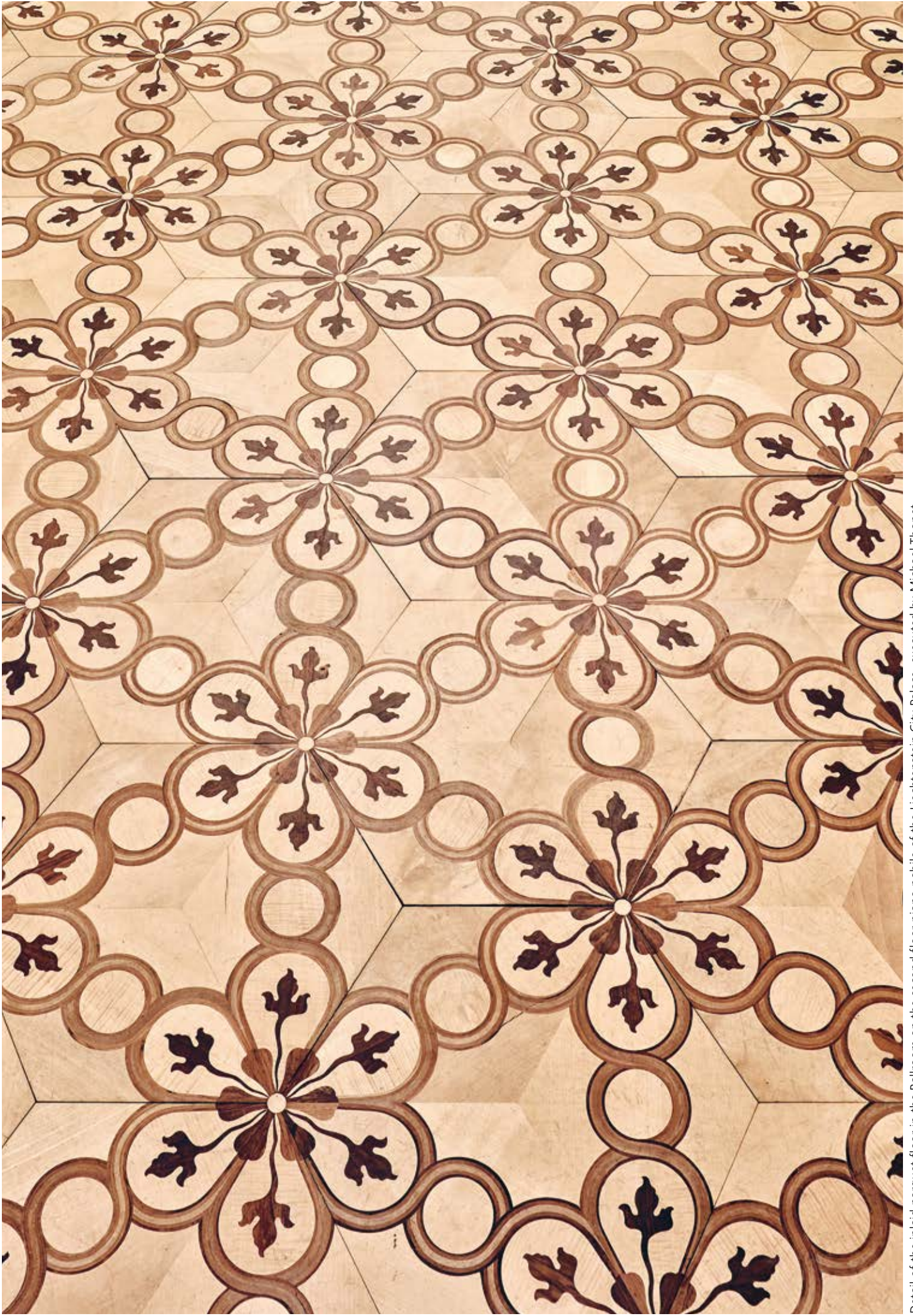
Detail of the inlaid parquet floor in the Ballroom on the second floor piano nobile of the Liechtenstein City Palace, executed by Michael Thonet
