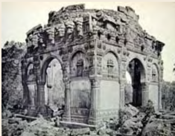
Mausoleum near Nagina Masjid : Before and after conservation by ASI
