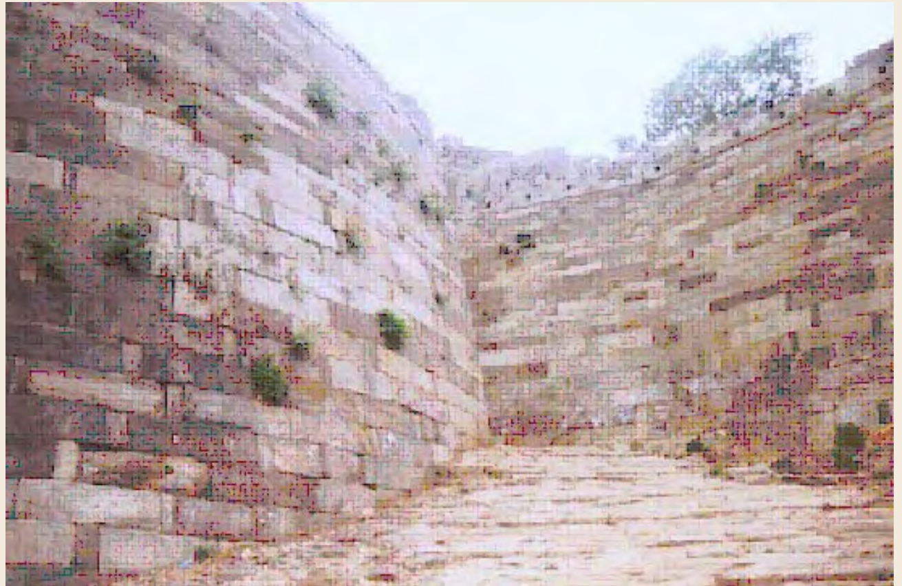
Sadan Shah Gate: a paraboloid entry into the Rajput fortification
