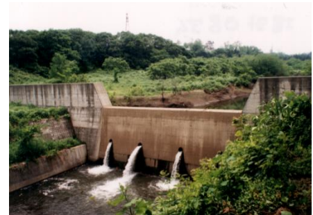
Sand control dam
