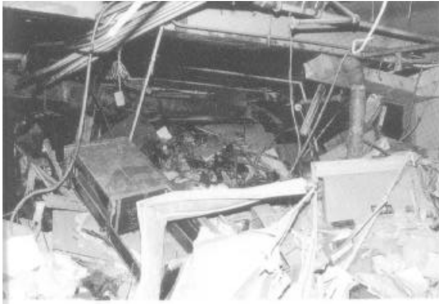
This destroyed office area on the B-2 level is typical of the debris piles faced by searching firefighters. (Photo courtesy of Port Authority Risk Management.)
