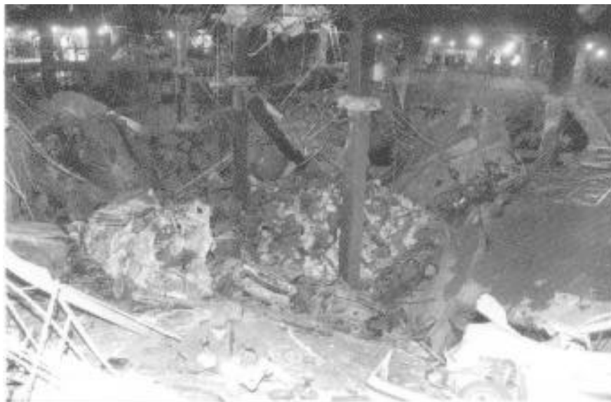
The crater, looking from the B-2 level down to B-5, taken during the investigation/restoration phase. (Photo courtesy of Port Authority Risk Management.)
