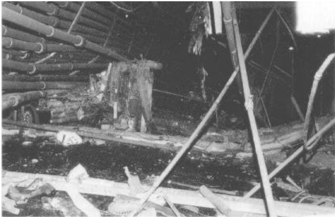
Building systems in the vicinity of the blast were destroyed. Here, twisted electrical conduit has landed on top of what was once a car. (Photo by FDNY Photo Unit.)
