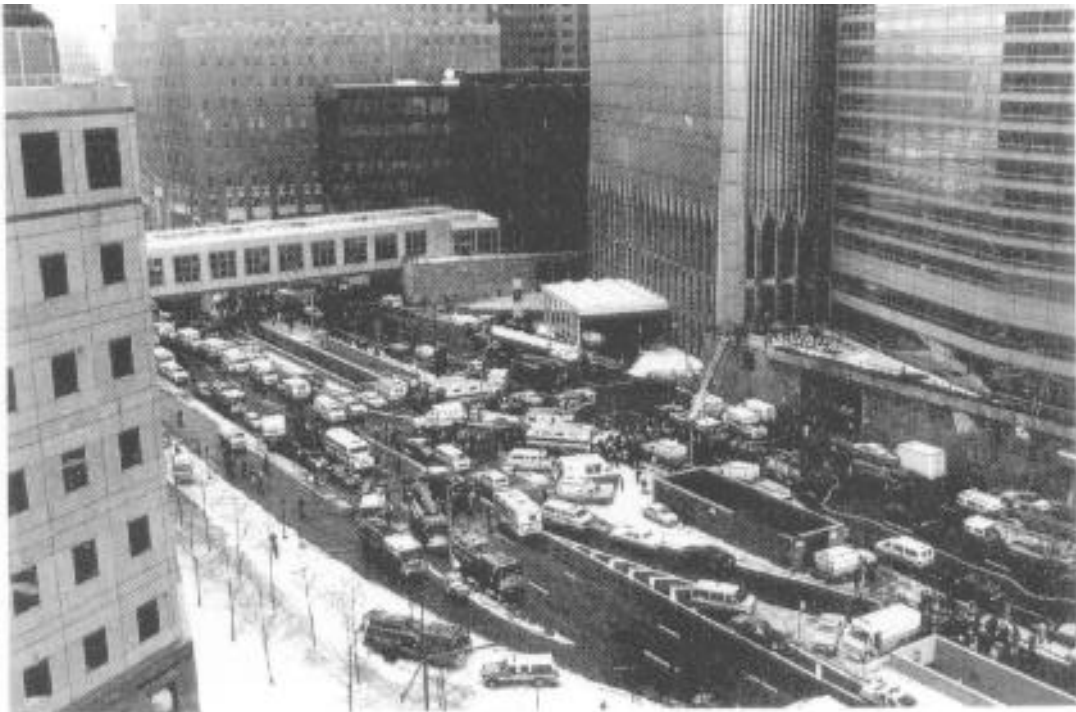
The scene on West Street within the first hour of the incident. The Vista Hotel is to the far right, and Tower 1 is next to it. The parking garage entrance is visible. Note also the tower ladder raised to the plaza level to remove occupants trapped at that level. (Photo by FDNY Photo Unit.)
