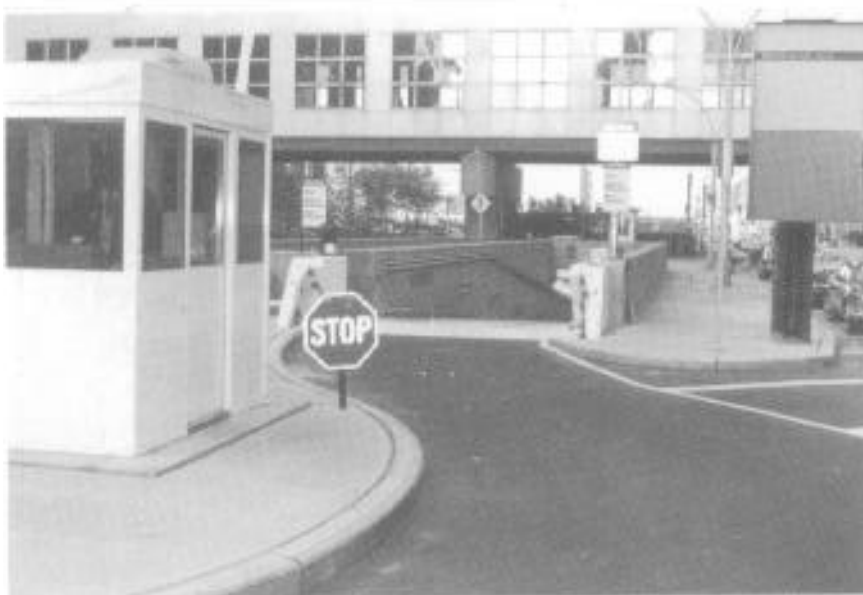
Controlling access to public buildings is a major concern for building management. After the incident, Port Authority, in addition to many security changes, installed substantial barriers to unauthorized vehicle access. The barrier, controlled by security personnel in the booth, folds down when the driver has been cleared to enter. (Photos courtesy of Port Authority Risk Management.)
