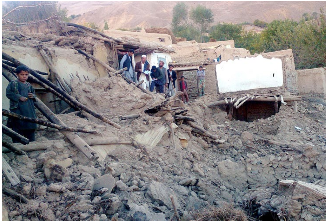
Aftermath of October 2015 earthquake in Badakshan province, Afghanistan. (photo courtesy of the International Organization for Migration)
