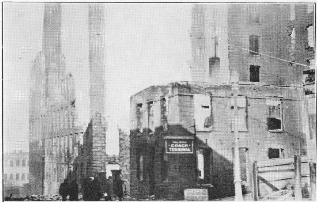
Pocasset Mill. South entrance of Bus terminal.
