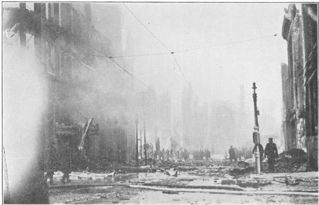
North Main St. looking south from Bank St.
