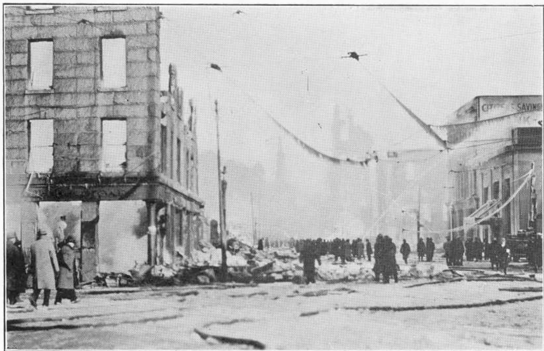
Main Street, Granite Block ruins on left. (Brady's corner.)
