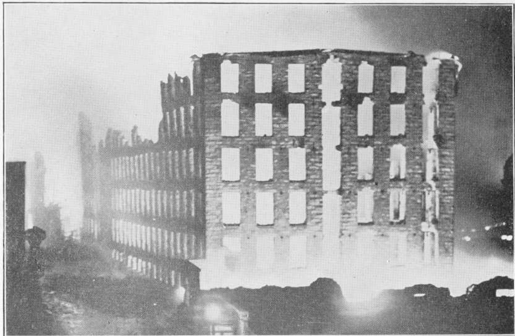
Pocasset Mill at the height of the fire.
