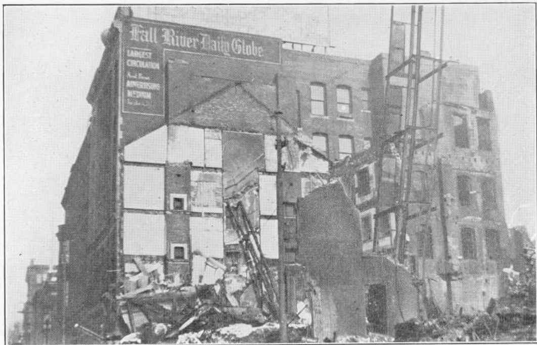
Fall River Globe Building. Fire Wall and Water Curtain saved this building.
