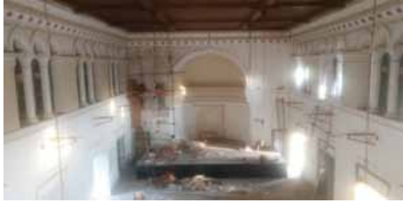
Ongoing work at Town Hall
