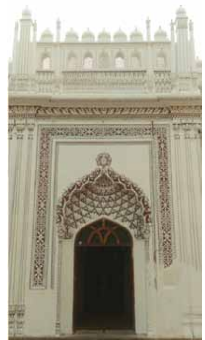
Conservation work nearing completion
