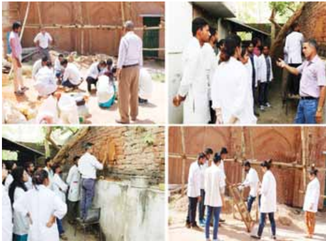
Participants working on project site on dummy wall
