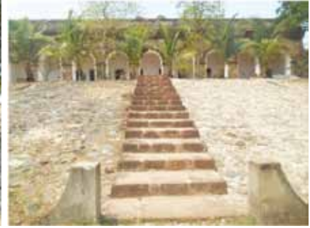
Hukitola building: after restoration
