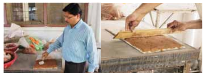
Application of plaster using trowel
