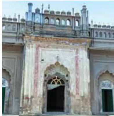
Shabi Mosque except for front façade, repaired in cement
