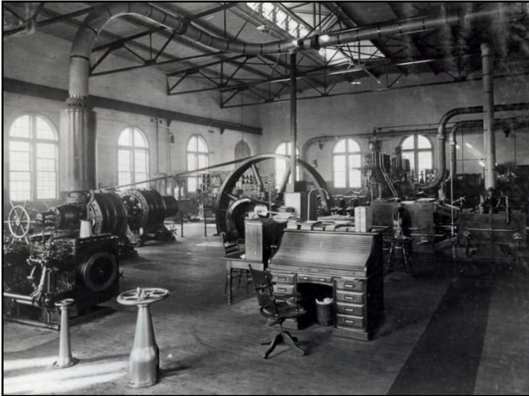
The GE transformer plant in Pittsfield, Mass, about 1900; the power station with 2-phase 2.3 kW belt-driven generators driven by reciprocating steam engines
