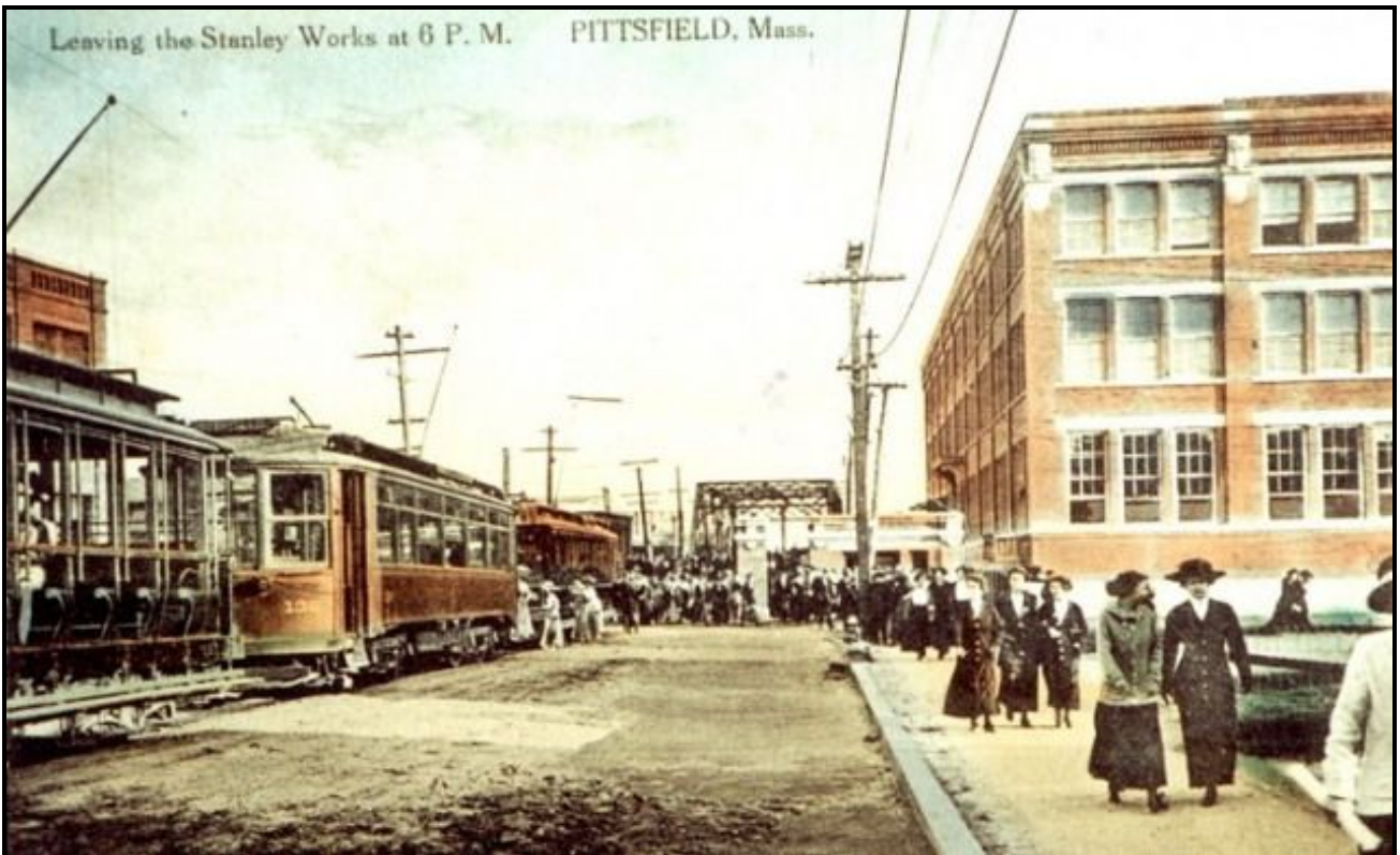
The Pittsfield Works in 1913
