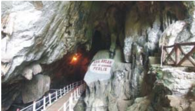
Figure 18a. Some basic infrastructures built in Gua Kelam to support tourism industry.
