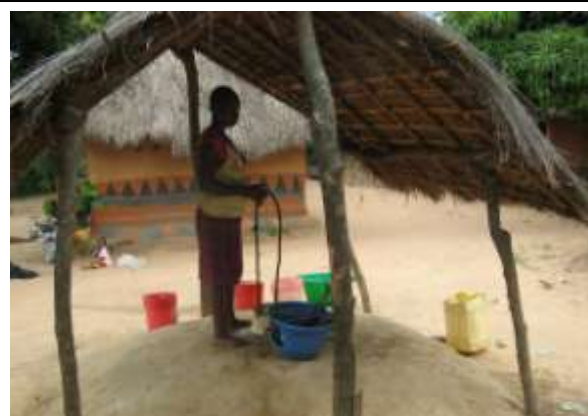
First stages of improvement in Nchelenge, stopping surface and rainwater running in. Keeping the rope clean
