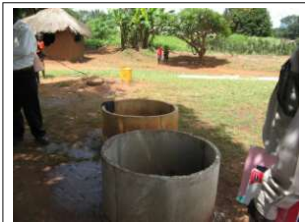
Sila Mumba's first two rings with the unimproved traditional well behind. He started the trend.
