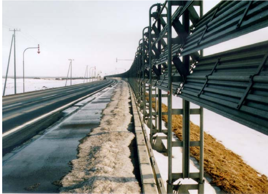
FIGURE 1 Blower snow fence equipped with angled fins that redirect wind downward to prevent snow from suspending the driver's line of sight.
