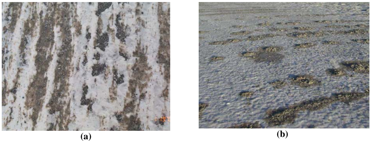
FIGURE 5 Road surface textures: (a) roller distributor and (b) spinner.
