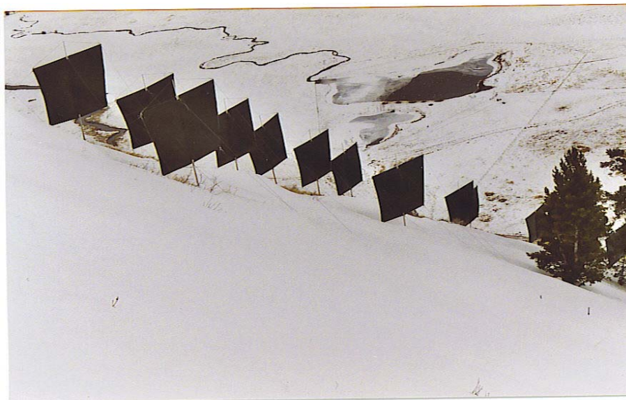
FIGURE 7 A view of a portion of the full snow-sail deployment of the 151 avalanche.
