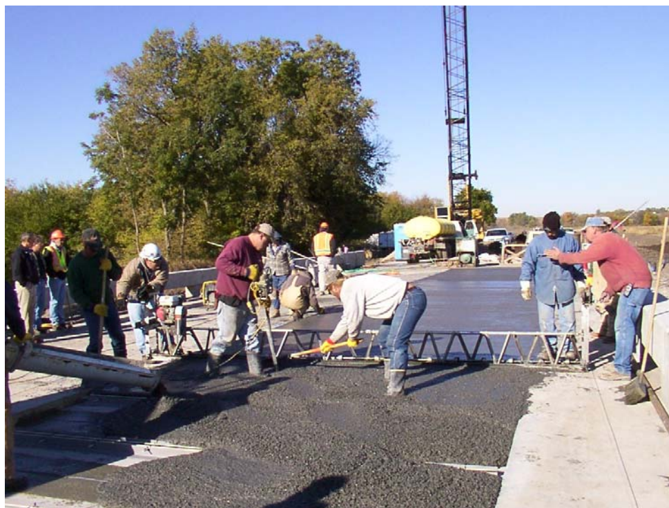
FIGURE 9 Casting the westbound lane with conductive concrete.
