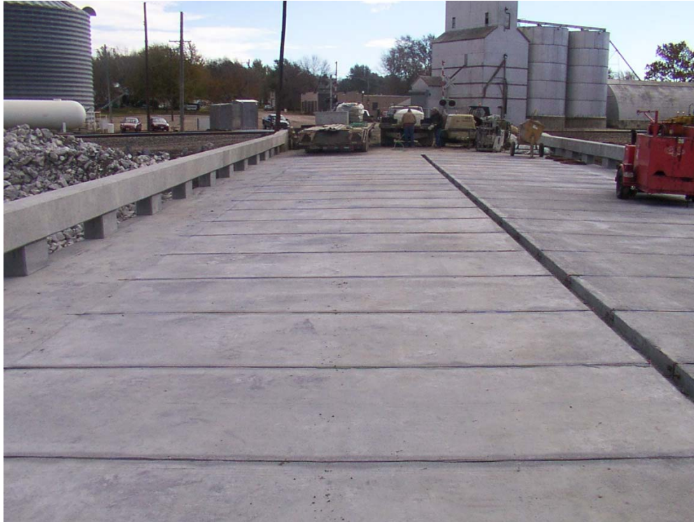
FIGURE 11 Total of 52 slabs after saw cut the inlay.
