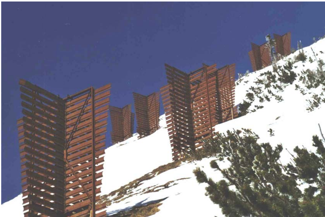
FIGURE 2 Modern European technology trails with omni (wind) directional kolkalfen in the Austrian Alps.
