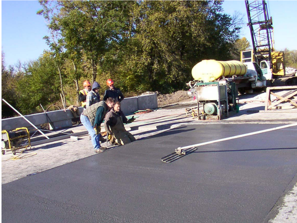
FIGURE 10 Finishing the conductive concrete inlay.
