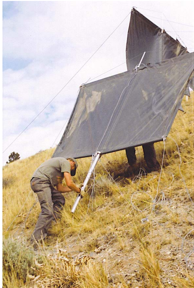
FIGURE 4 Personnel reinstalling one of the 50 sails in the 151 avalanche full snow-sail deployment.
