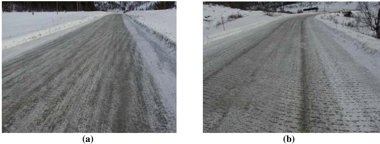
FIGURE 4 Typical pattern using warm wetted sand: (a) roller distributor and (b) spinner.
