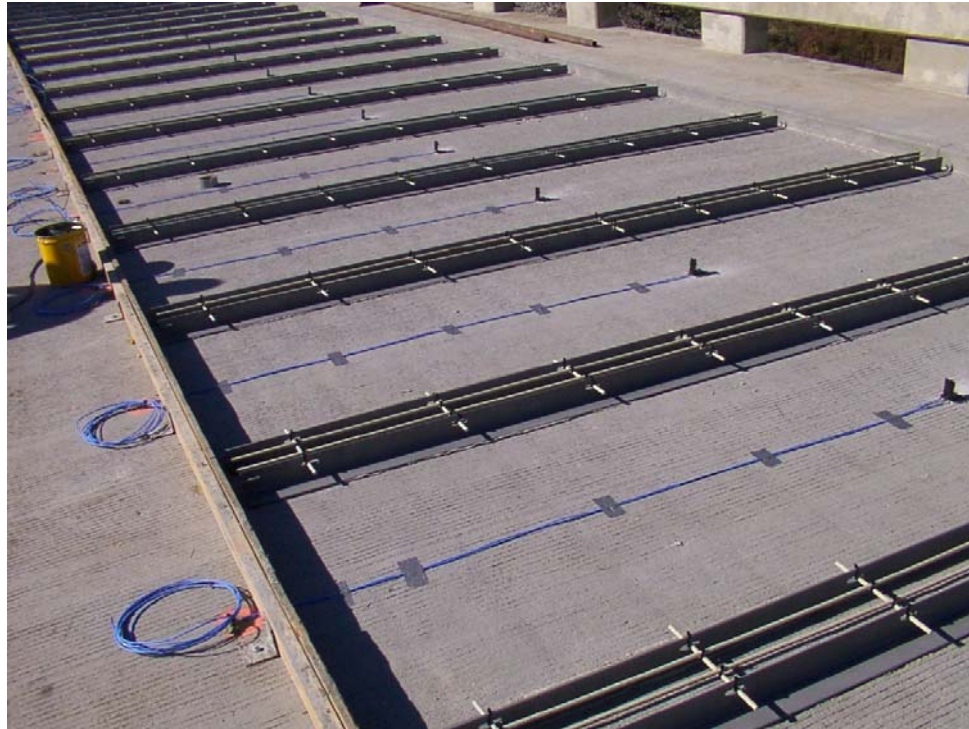
FIGURE 8 Electrode layout during construction.
