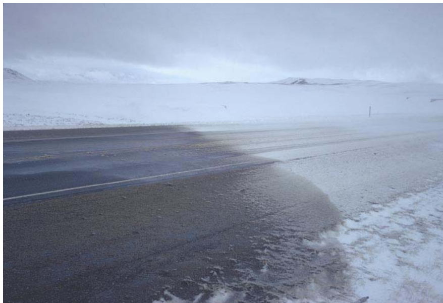
FIGURE 13 This transition from frozen slush to wet pavement corresponding to the beginning of the area protected by a 3.8-m-tall (12.4-ft) snow fence located about 150 m (500 ft) upwind.
