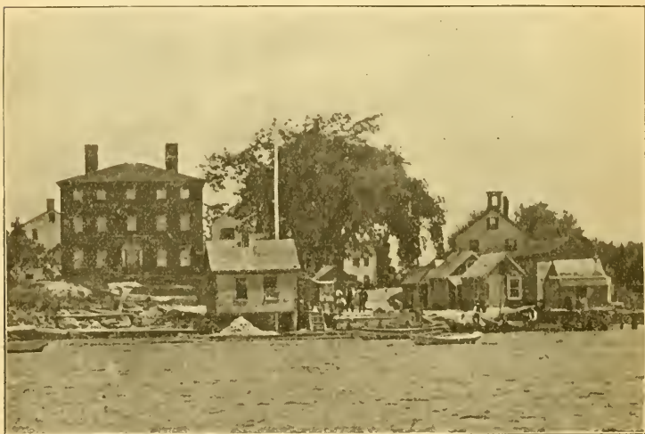
MARCH'S FERRY LANDING PLACE, SALISBURY SIDE.
