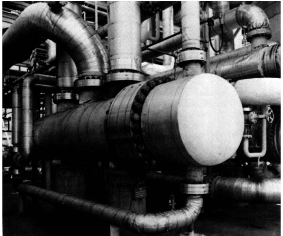
Type 304 stainless steel tubing extends heat exchanger service life in hydrogen production. Photograph: Union Oil Company of California
