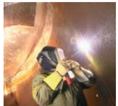
Refurbishing under way at Beauharnois generating station.
