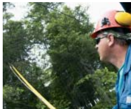
Pruning operations to prevent power failures.
