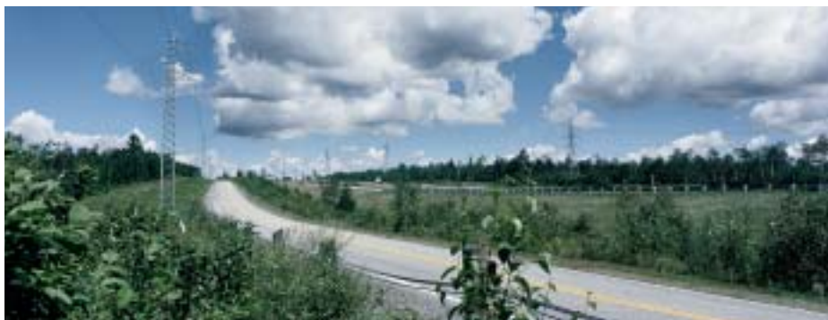
The new 120-kV line in the Magog area: harmonious integration with the landscape.
