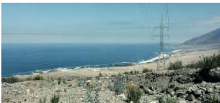
The Transelec transmission system, in Chile, is operated by Hydro-Québec TransÉnergie.
