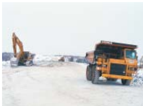
Construction of the access road for the Eastmain-1 project.
