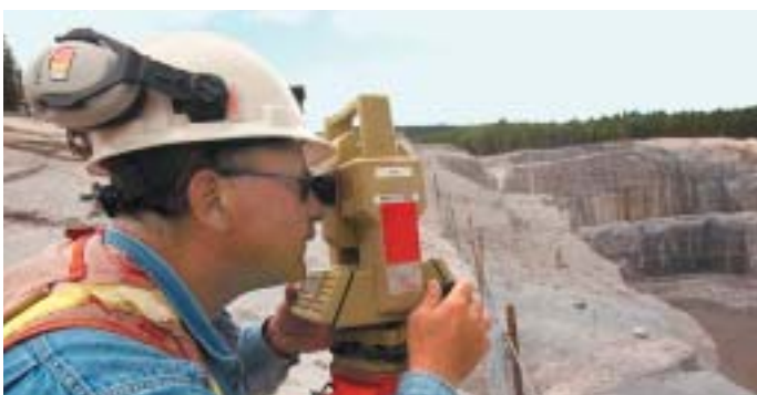
Surveying on the site of Toulnostouc generating station.
