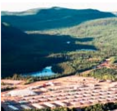
Construction of Toulnostouc generating station: the work camp.
