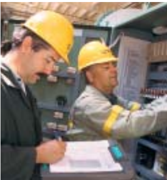
Workers finish refurbishing Shawinigan-2 generating station.
