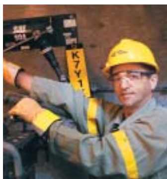
In downtown Montréal, work goes on to ensure compliance of the underground distribution grid.
