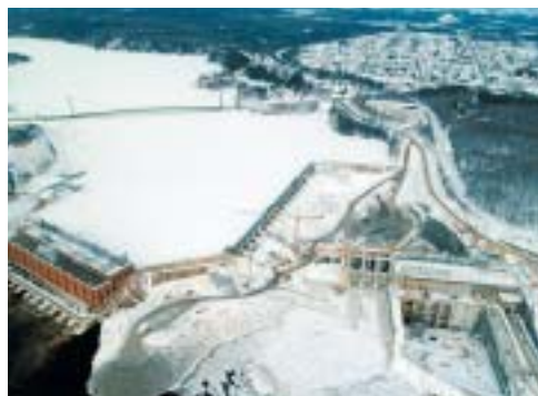
The new Grand-Mère generating station, a jobsite in an urban setting.
