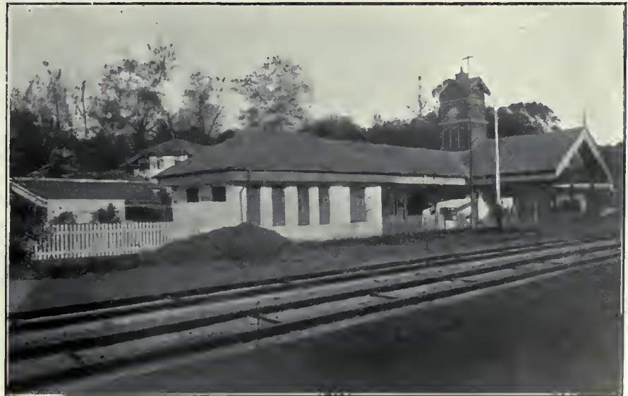
TANK ROAD STATION, SINGAPORE.
