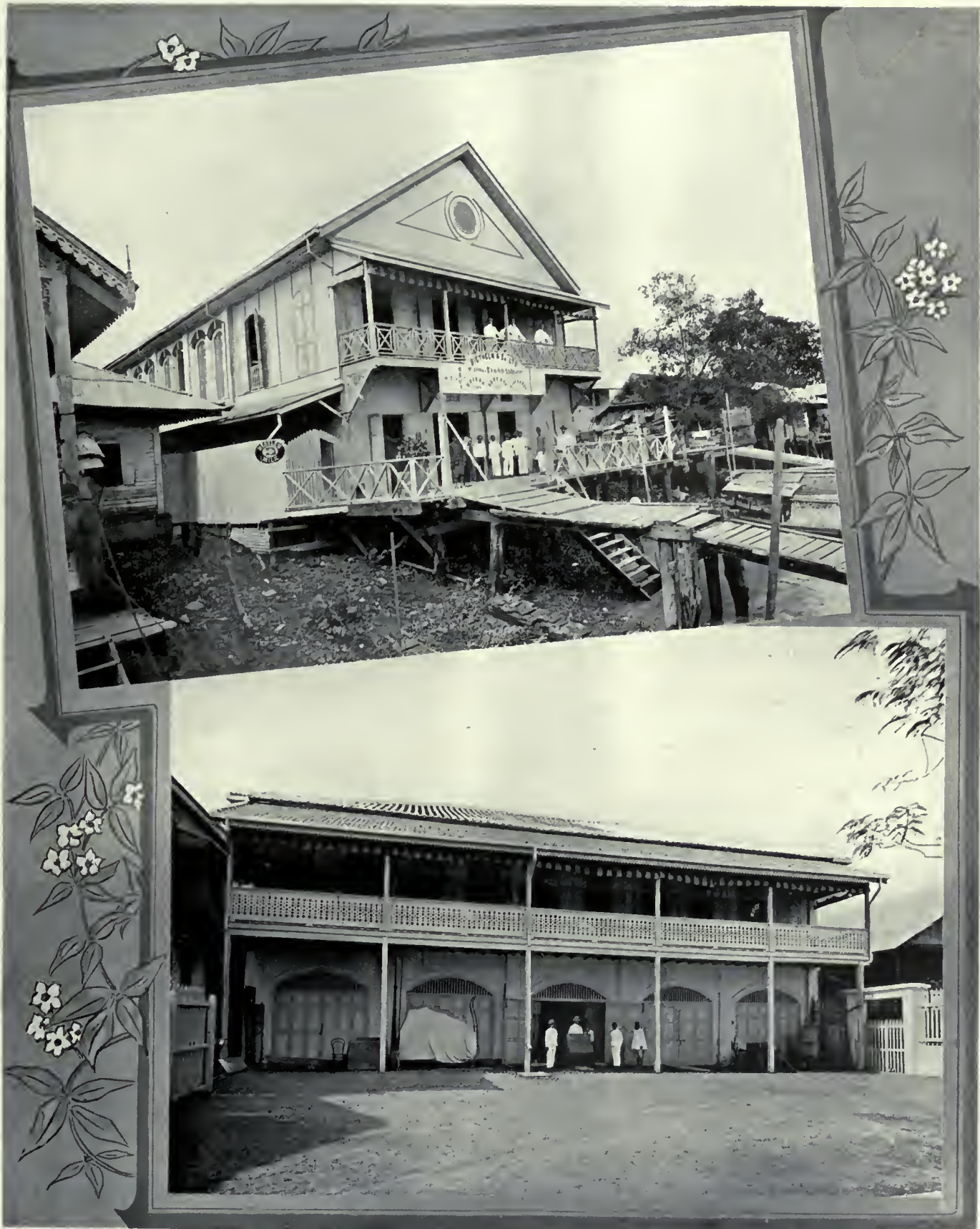
OFFICES AND GODOWNS OF MESSRS. DIETHELM & CO., LTD.
