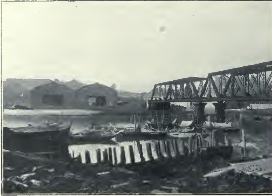
RAILWAY BRIDGE OVER SINGAPORE RIVER.
