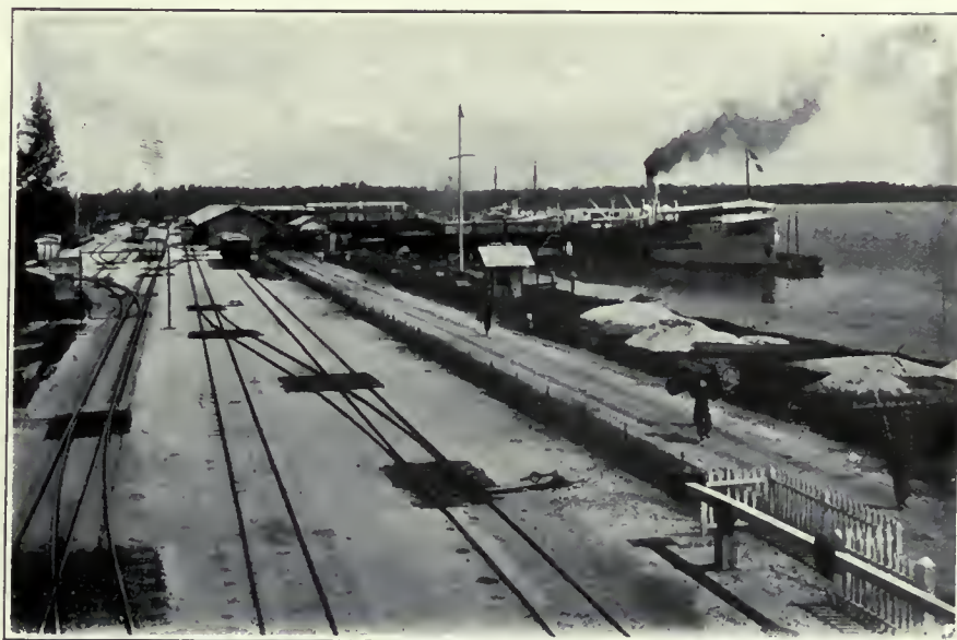
PORT SWETTENHAM—THE RAILWAY SIDING.
