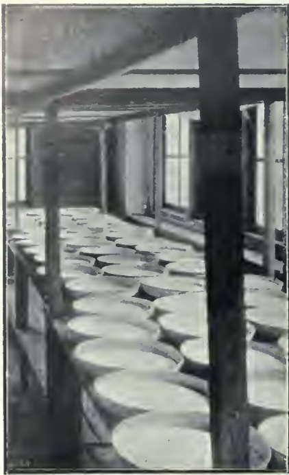
LATEX IN SETTLING OR COAGULATING PANS.
