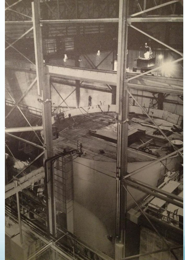
Hull and shield tank for the S1G prototype
