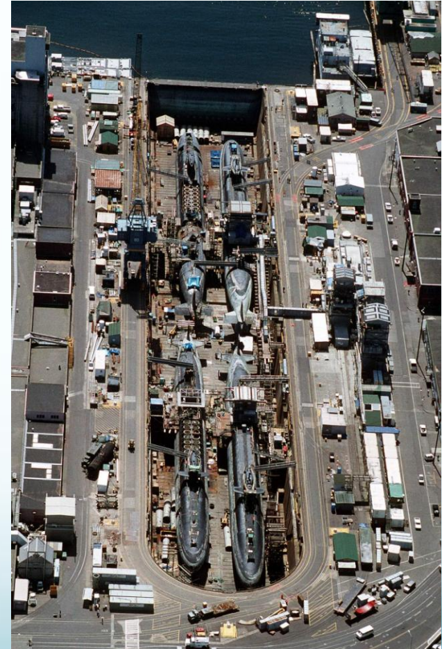
Four Lafayette class (SSBN-616) in the early stages of being scrapped at PSNS in 1993
