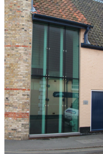
Fig 2: Example of Frameless Glass Façade with Stainless Steel Fittings and Mild Steel
