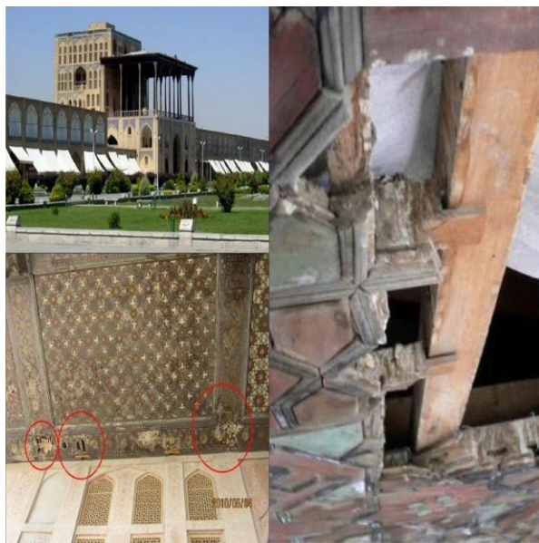
Figure 5: Increasing Emissions of Corrosive Acidic Pollutants such as Sulfur Oxides cause of deterioration of Wooden Ceiling of Ali Qapu palace.
