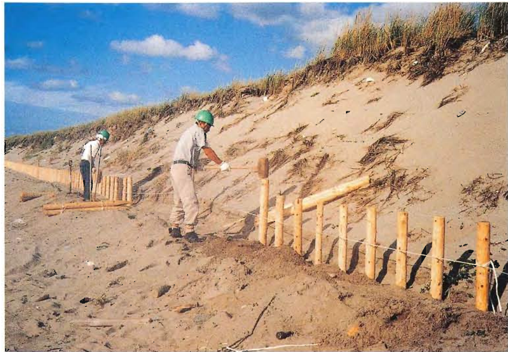
杭打込み0.5m間隔
